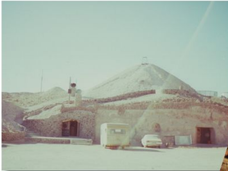
Left: Former Opal Dugout converted to Residence, Coober Pedy
